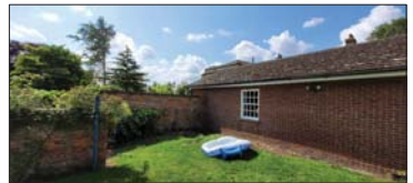
Photo of current wall prior to re-building of collapsed area
