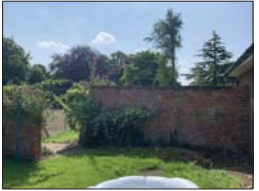
Photo of current wall prior to re-building of collapsed area
