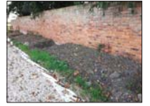
Photo of current drive / wall
