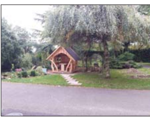
Photo of existing timber to be dark stained - dark oak stain
